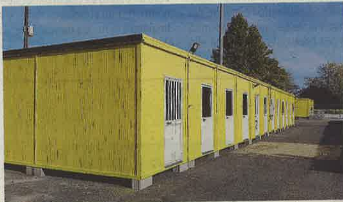
Container via Traves
